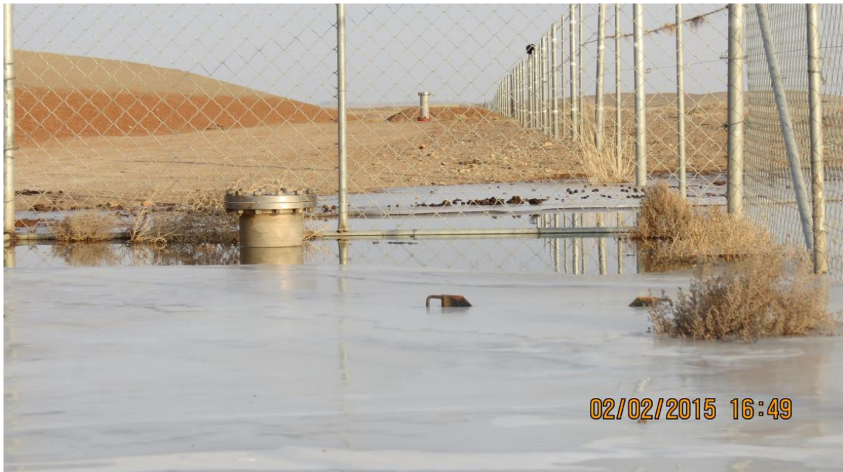
Figure 5.3: Inundation of Surface Flow Measurement Point by Ice Sheet
