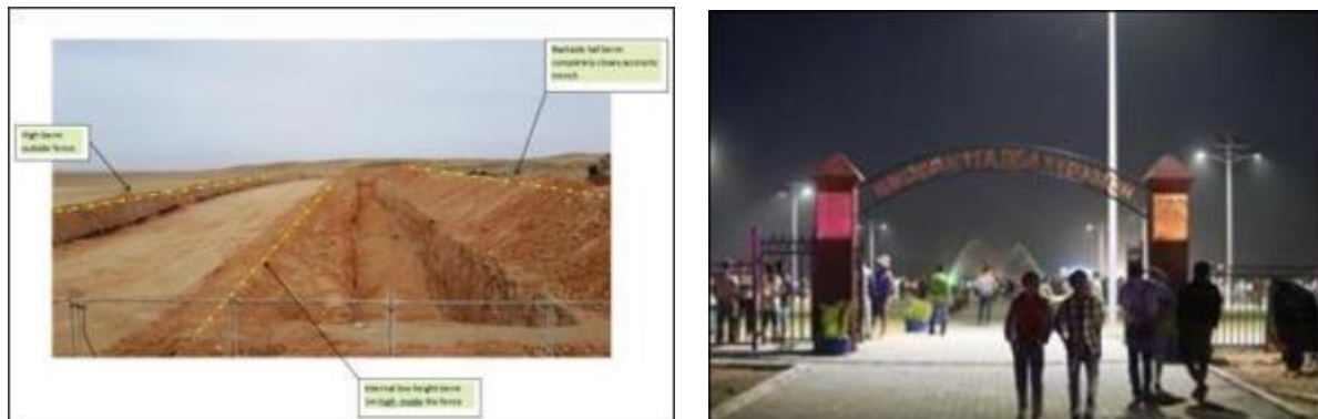
Figure 6.5: Interim Waste Facility Trench Work and Khanbogd Public Park (“Galba” Park)
