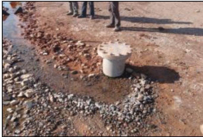
Figure 1: Outfall bore - diverted groundwater migrating up the gravel pack
