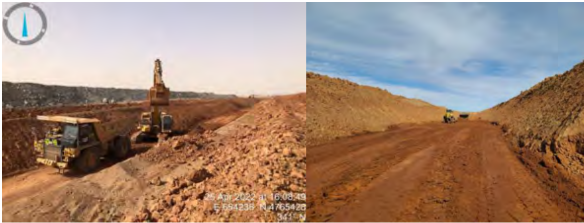
Figure 4-21 TSF Cell #2 Excavation for Clay Cut-Off Trench (up to 12 m below surface)
