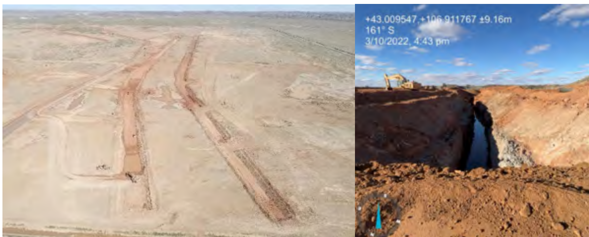
Figure 4-23 Aerial View of TSF Cell #2 Cut-Off Dam (left) and Seepage Collection Trench (right)
