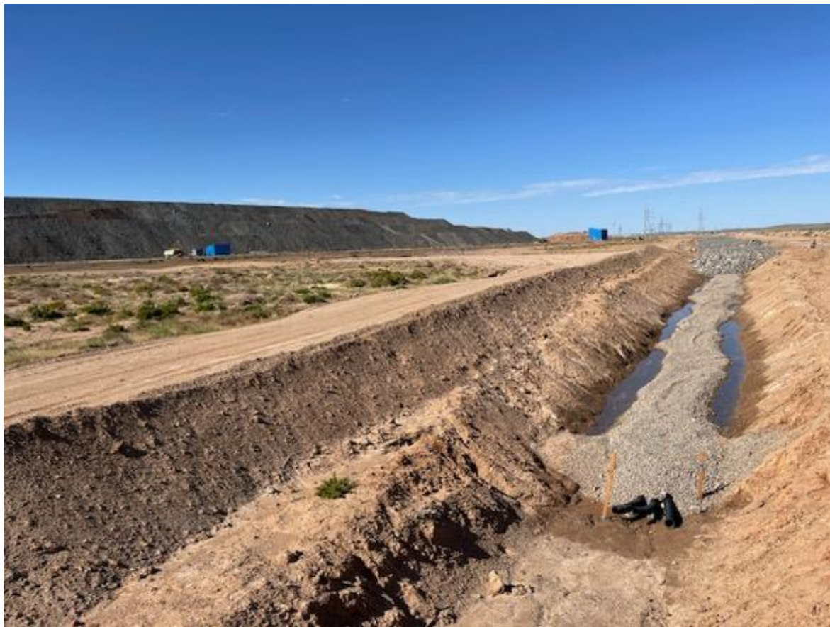
Figure 4-32 Installed French Drain System (to be covered)
