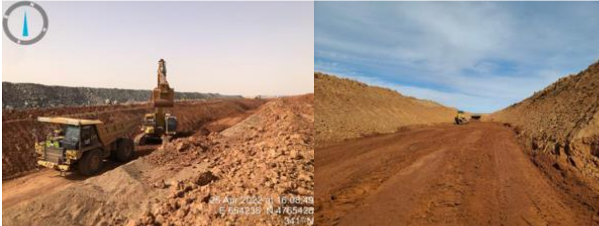
Figure 4-34 TSF Cell #2 Excavation for Clay Cut-Off Trench (up to 12 m below surface)
