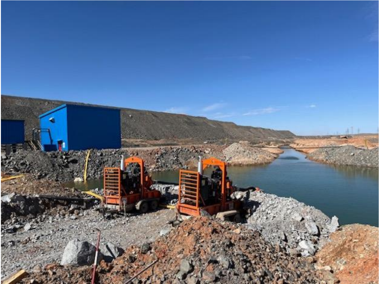
Figure 4-33 Relocated Seepage Collection Pump House and Seepage Collection Pond
