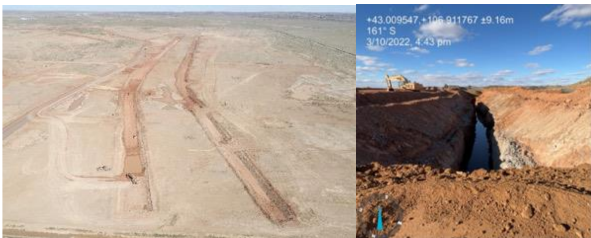
Figure 4-36 Aerial View of TSF Cell #2 Cut-Off Dam (left) and Seepage Collection Trench (right)
